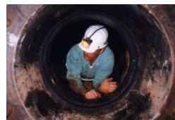
Install Rubber Seal
