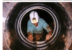
Install Retaining Bands
