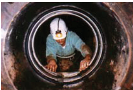
Install Retaining Bands
