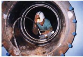
Expand Bands with Expander
