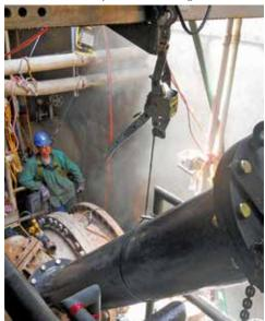
tic and catalyst line that had complete joint failure. Tight working conditions prevented use of bulky conventional line stop equipment. The unit could not be shut down. The 150 psi line required a plug that could handle 300 psi inflation pressures.
