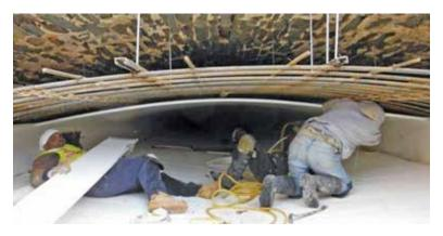
contractor, Boyer Inc., had the reinforced steel, liner, numerous service connections and grout successfully installed ahead of schedule.
