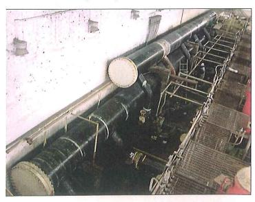
installation. The new wrap product is qualified in accordance with ASME Standard Post construction Test (PCC-2) as well as other governing documentation. All installers must complete classroom training and hands-on application training prior to installation in the field.
