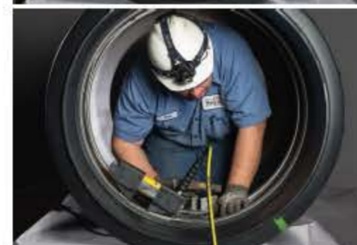
Expand Bands with Expander
