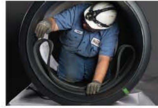
Install Rubber Seal
