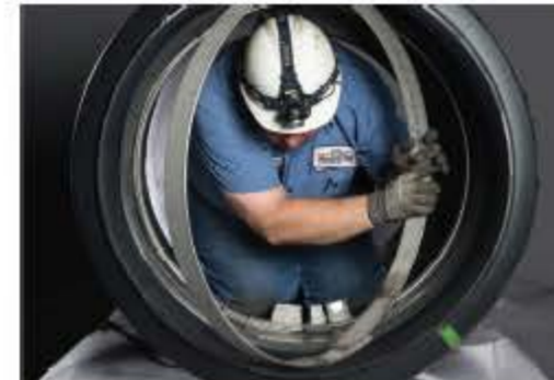
Installing Retaining Bands
