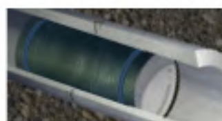
9. Deflate Packer & Remove it from the Pipe
