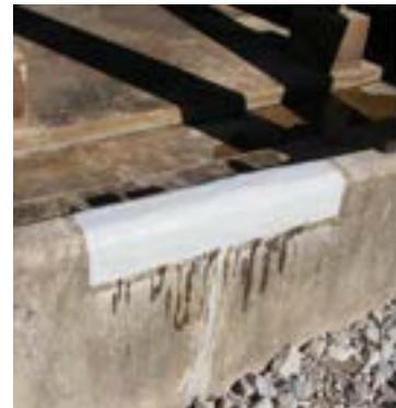
The joint transition in the cooling tunnel had to be cleaned and leaks had to be drilled and then filled with hydraulic cement. Then this cement was used to contour and smooth out the abrupt transition. Once the prep work was completed, four layers of HydraWrap were installed. Once the HydraWrap had cured, a 70" diameter retaining band was installed on the 70" round side, on top of the edge of the HydraWrap. Eight flat bars were installed on the HydraWrap's other side.
