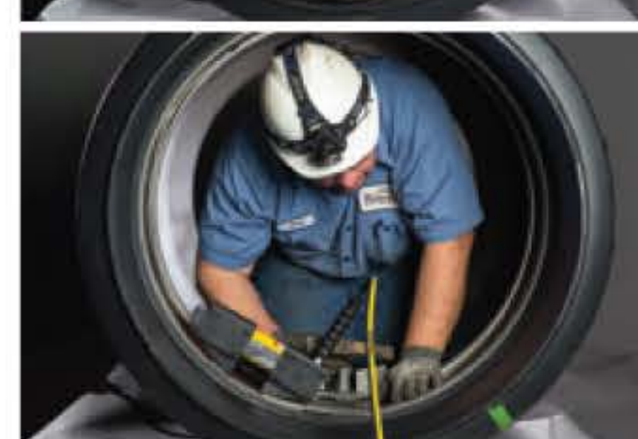
Expand Bands with Expander
