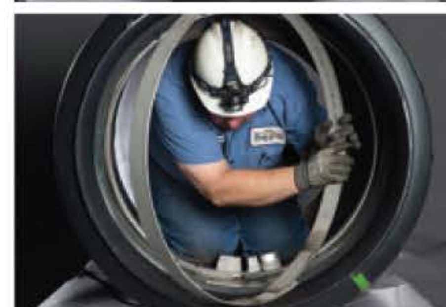
Installing Retaining Bands
