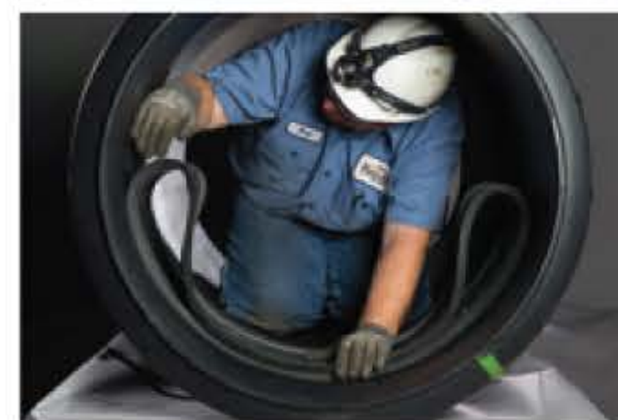
Install Rubber Seal
