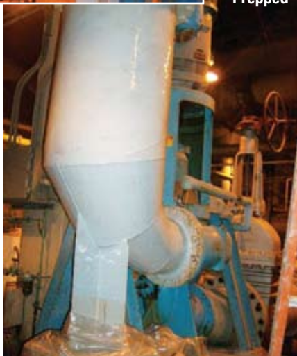
The reinforced composite system presented to the North Tonowanda facility is an alternative means to permanently repair leaks and arrest corrosion.
