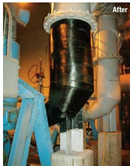
The reinforced composite system presented to the North Tonowanda facility is an alternative means to permanently repair leaks and arrest corrosion.
